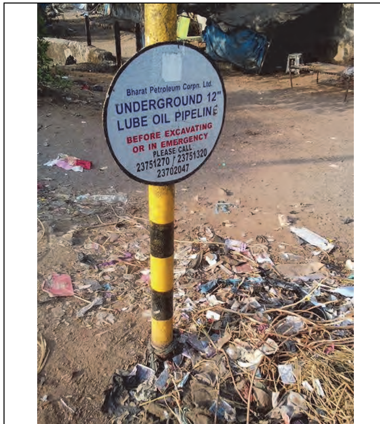
Figure 6 BP LUBE Oil pipe line at Sewri side
