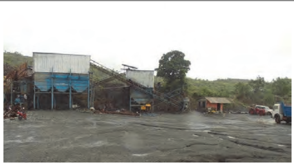
12: ROW (rock & sand crashing plant)
