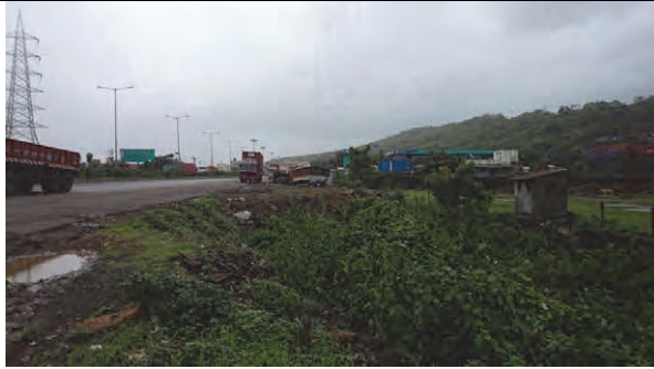
19: road crossing point with JNPT highway <toward N>
