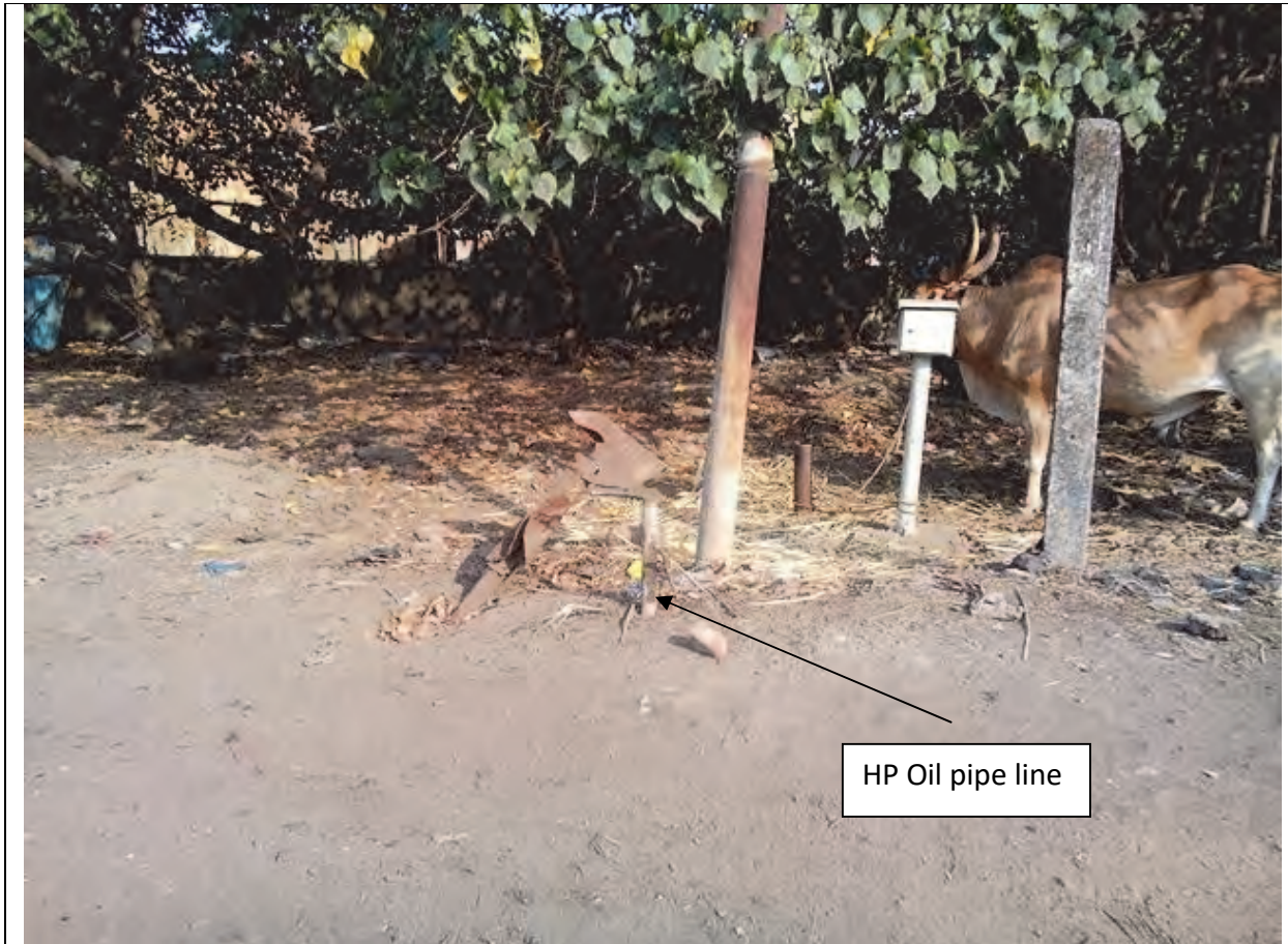
Figure 5 HP Oil pipe line at Sewri side
