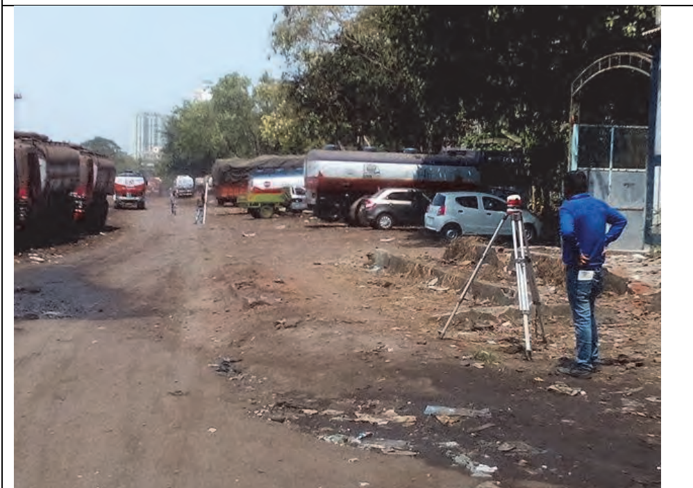
Figure 8:-topographic survey work at Seweri Site
