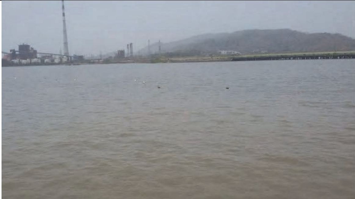
Figure 18 Pir Pau Jetty at KP5.88
