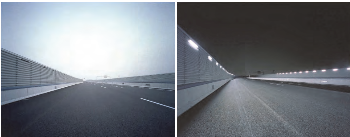
Figure 12.4.8 Noise Barrier with Lighting System in the handrail/noise barrier/view barrier
