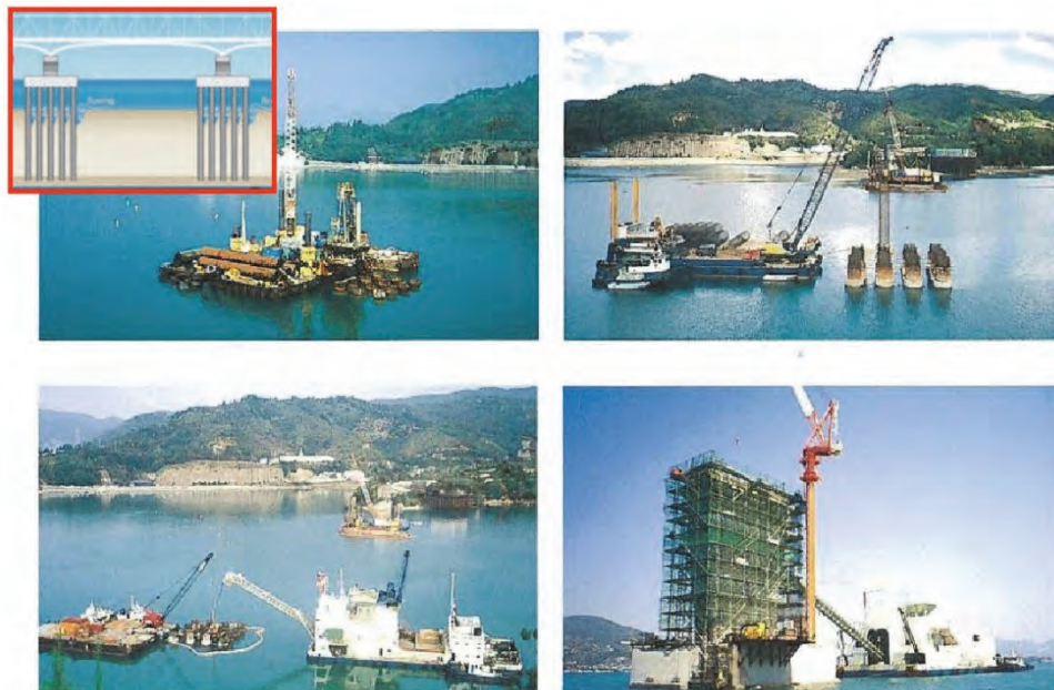
Figure 12.4.6 Bored Piling Methodology for Prevention of Turbid Water
