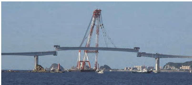
Figure 7.2.15 Large Block Erection Method Using Floating Crane
