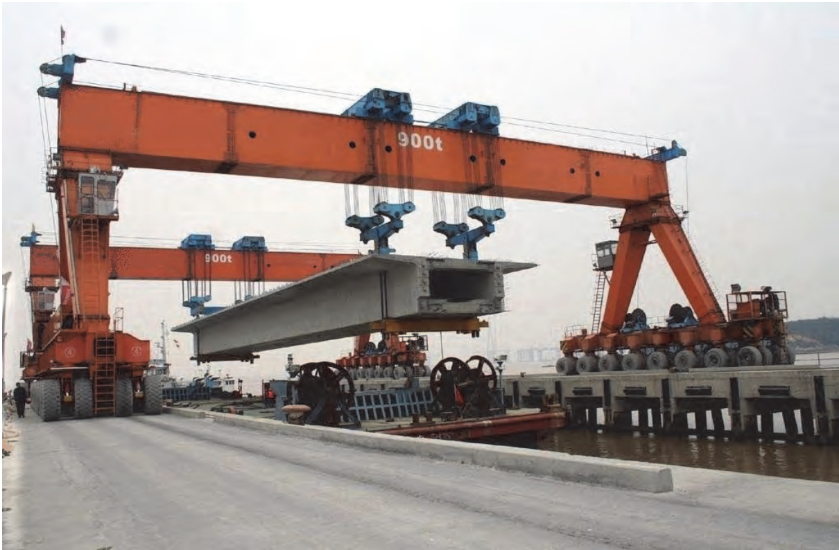
Figure 7.2.17 Full Span Erection Method (Using Gantry Crane)
