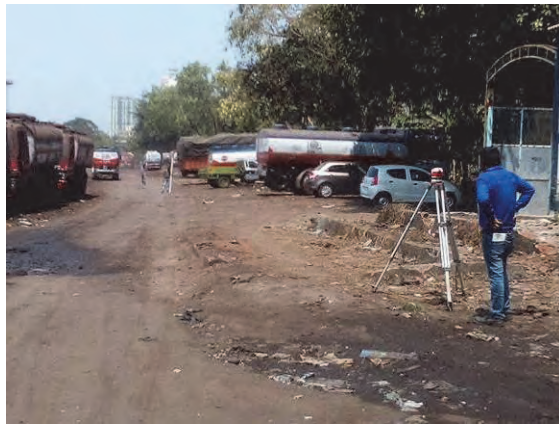
Topographic survey work at Seweri site
