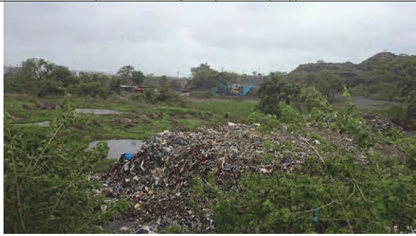
7: Land Fill(front) & Unused land in ROW(far) <toward NW>
