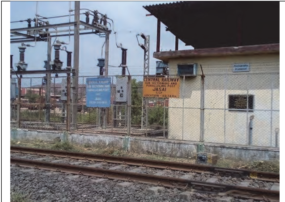
Figure 10 Railway line at Jasai crossing the MTHL alignment and electric transformer
