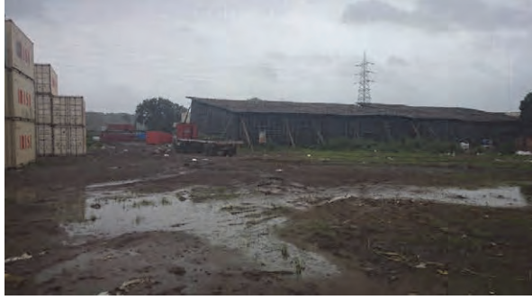
17: ROW (temporay storage) <toward E>
