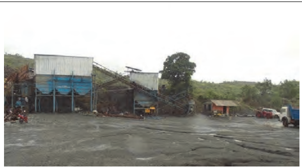
12: ROW (rock & sand crashing plant)
