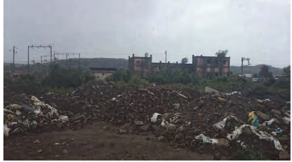
16: ROW (abandoned buidling and railway track) <toward W>
