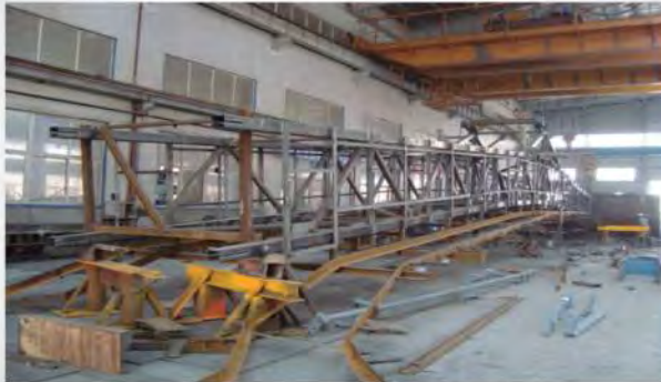
Earlier condition of the structural work shop (2009.04.09)
