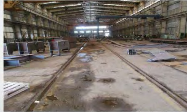
Structural work shop at present (2016.04.16)
