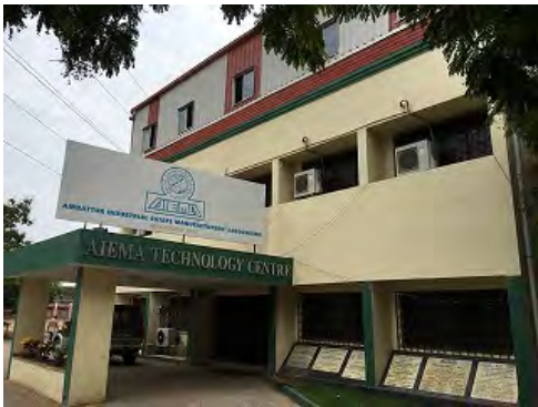
▲ AIEMA Technology Centre building
