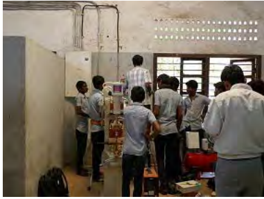
▲ Trainees being mobilized for electrical works
