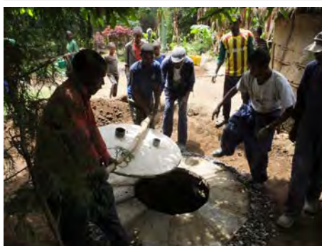
Placing of well cover 4
