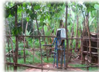
Pump located in the middle of farmland
