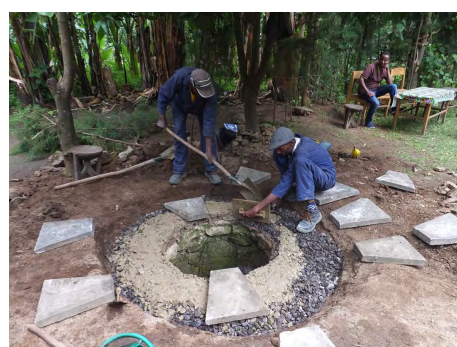
Setting of reducer blocks 2
