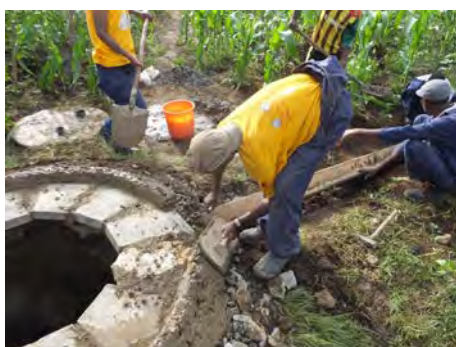
Construction of apron, drainage canal and soak away pit 3
