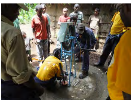
Installation of Rope Pump 7
