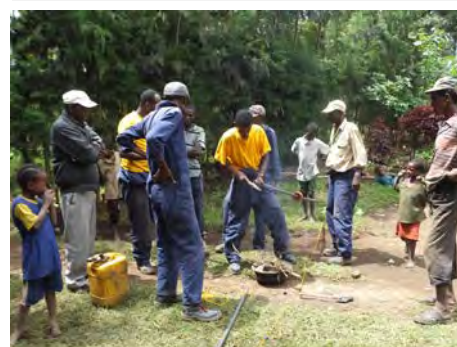
Preparation of riser pipe, rope and pistons 5
