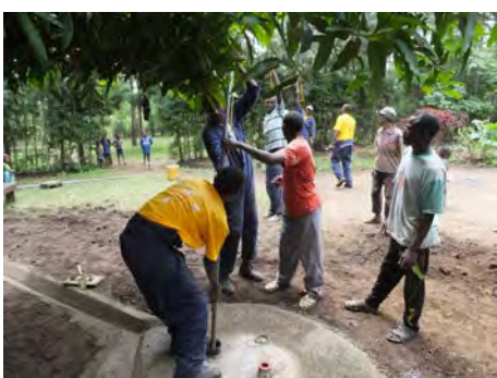
Installation of riser pipe 6
