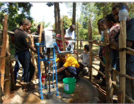
Pouring high chlorine dissolved water into the well
