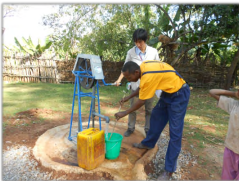
Zerihun (yellow T-shirt), from Dale Woreda Water Office, is mixing chlorine before putting to the well.
