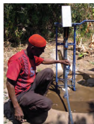
Attache a funnel and a hose to outlet of RP
