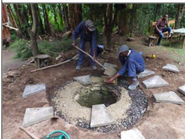
Installation Training for Village Technician ( May 2015, Damot Pulasa )
