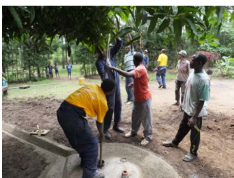
Installation of riser pipe 6
