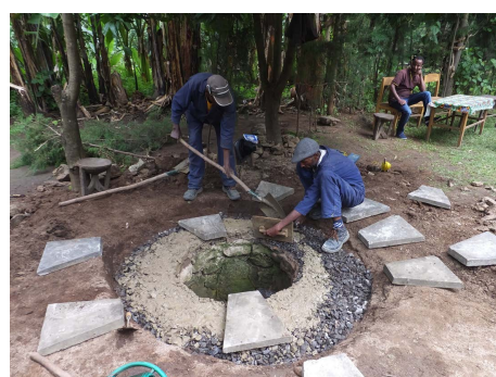
Setting of reducer blocks 2
