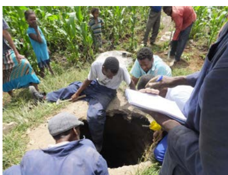
Measuring of depth and water level of well and checking well structure before installation of Rope Pump. 1
