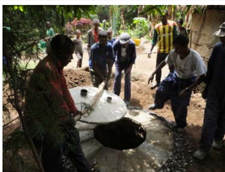
Placing of well cover 4
