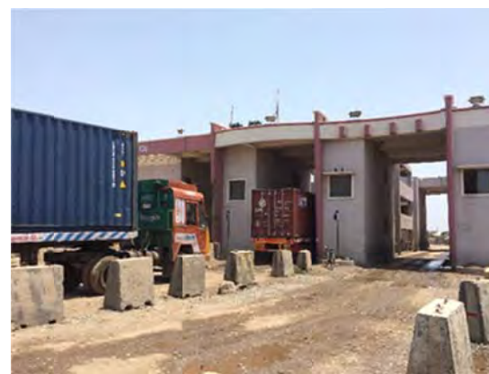
Picture 3-9 RFID Reader around Exit of Port Gate No.1
