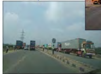
Traffic Control at SH 114
