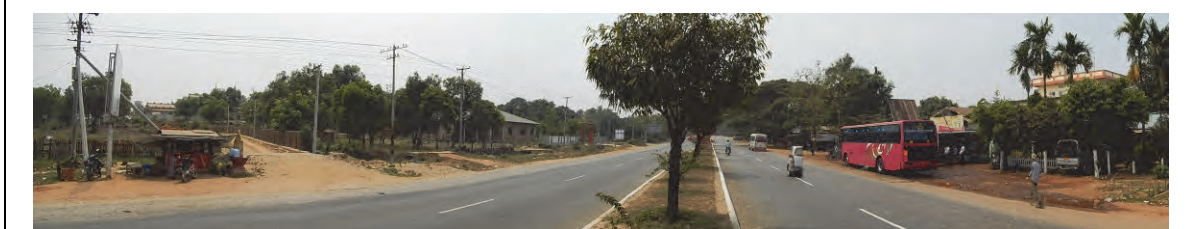
Current state of the roadside of NH-1 where the structures may be affected in the Bago region
