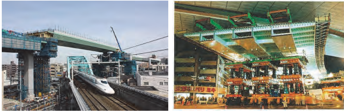
Figure 7.2.9 Example of Erection by Launching Erection Method (Left) and Multi-Axle Truck(Right)
