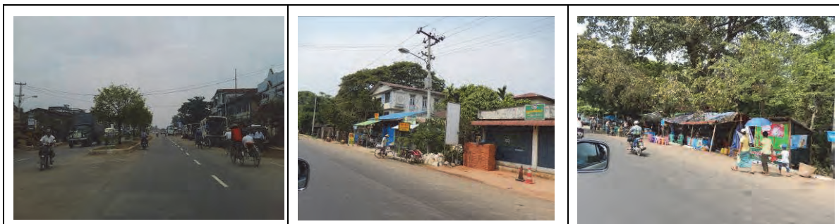
Current state of the roadside of NH-1 where the structures may be affected in the Yangon region
