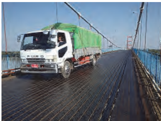
Photo-16 Gyaing Zathapyin (GZ) Bridge
