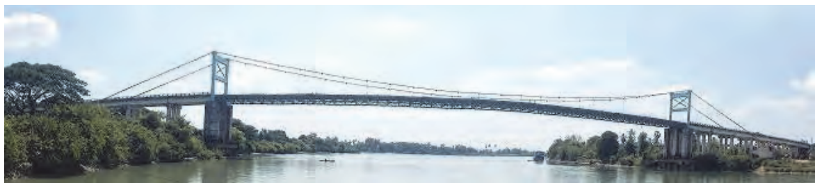
Photo-9 Gyaing Kawkareik Bridge (Existing)
