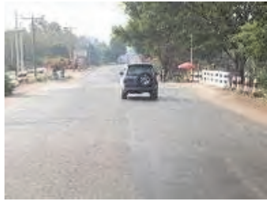
Photo-21 Road Condition on Mawlamyine - Thanbyuzayat
