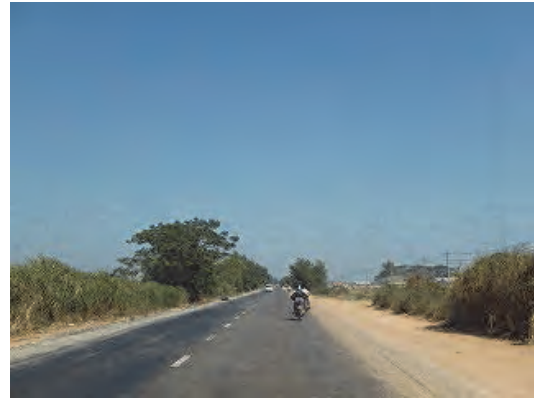
Photo-2 Road Condition on Bago – Payagyi Section
