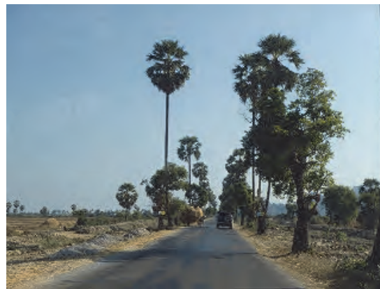
Photo-15 AT Road Condition on AT Bridge-GZ Bridge
