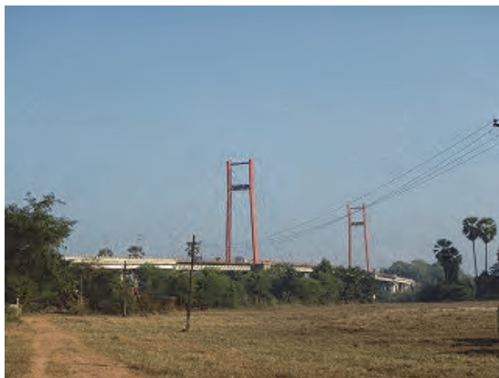
Photo-14 Atrán (AT) Bridge
