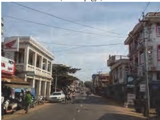
Photo-5 Road Condition at Kyaito
