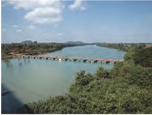
Photo-10 Pontoon Bridge
