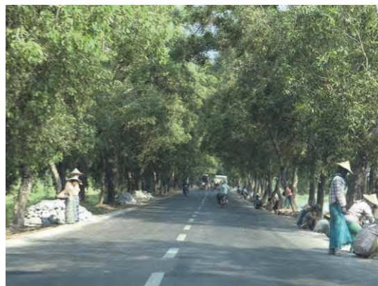
Photo-19 Road Condition on Zathapyin – Hpa-an
