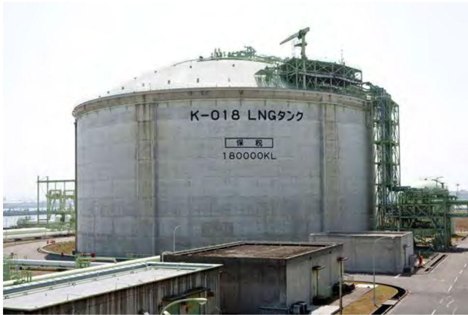
Figure 8-23 Overview of Above Ground Dome Roof Type PC LNG Storage Tank
