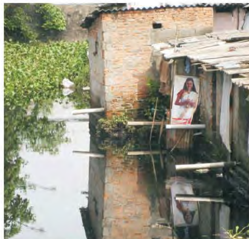
Figure 34: Clogging of storm drains
