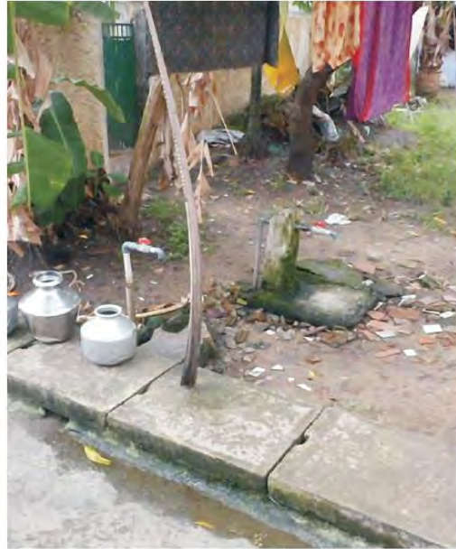
Figure 35: Poor service delivery of water supply
