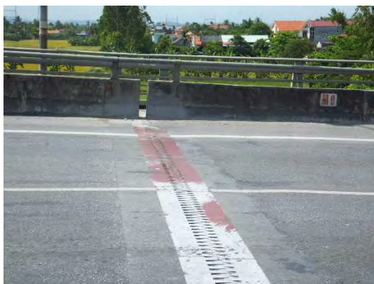
The expansion joints have been replaced by new ones.
