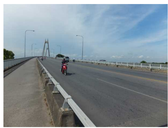
The south approach of Binh Bridge. The vertical gradient is 4%, which is the same as Kien Bridge.
