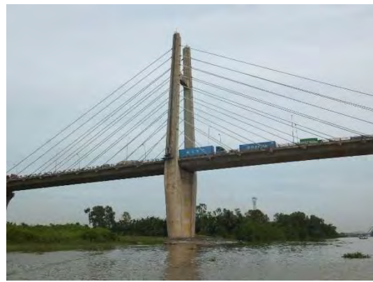
Large trucks pass on the deck.
