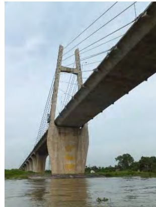
Concrete box girder and the north tower.
