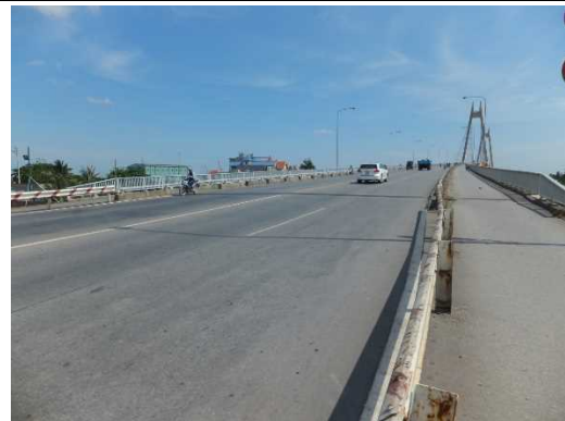
Binh Bridge has 4 lanes and a wide pedestrian walkway, about 4m wide.
