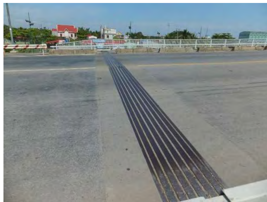
Expansion joint on the bridge.
