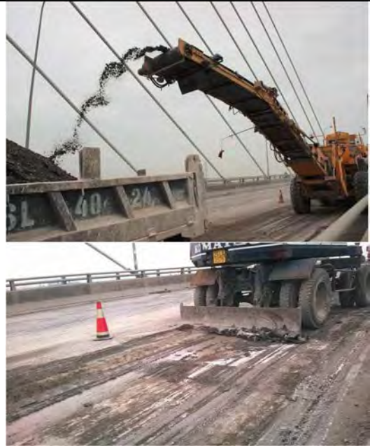
Repavement of Kien Bridge, November 2014 Source: http://www.baohaiphong.com.vn/ <03/09/2014>
