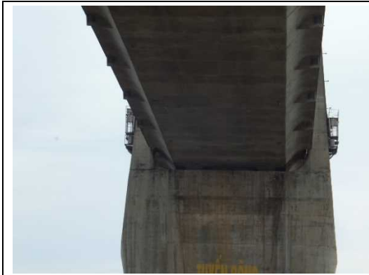
PC concrete box girder. The box girder is constructed from segments.
