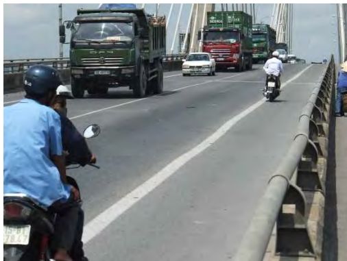
Heavy trucks keep passing on the bridge.
