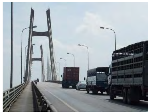
As heavy trucks are slower, traffic congestion is common. The vertical gradient of the bridge is 4%.
