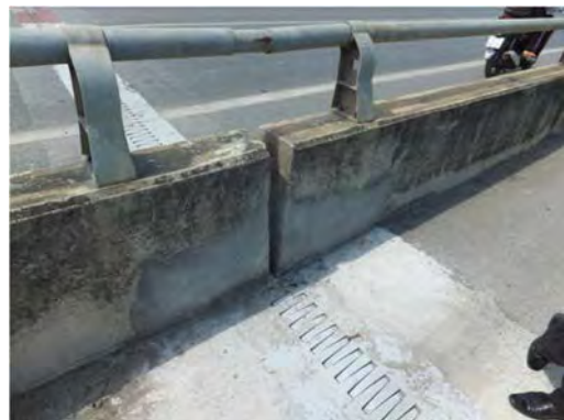
All of the expansion joints on Kien Bridge were replaced. The reason is unknown.
