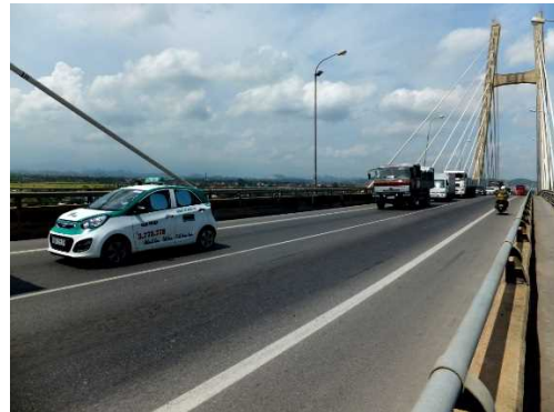
Heavy trucks keep passing on the bridge.
