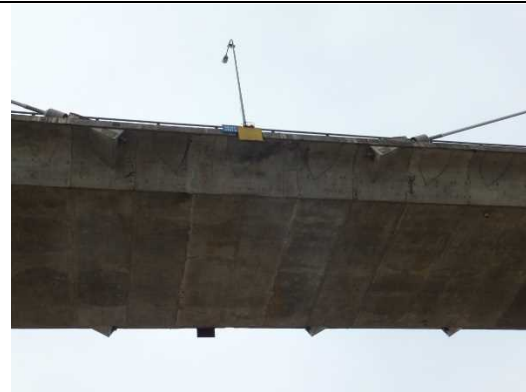
The center of the span. Cable anchor structures are visible.
