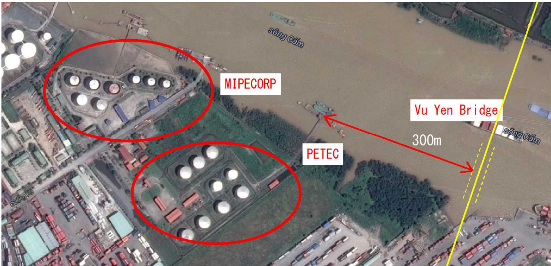
Figure 6.2-7 Oil Facilities near Proposed Location of Vu Yen Bridge
