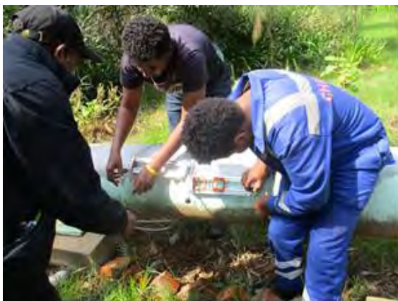
Figure 3-8 Training of Installation of Water Flowmeter
