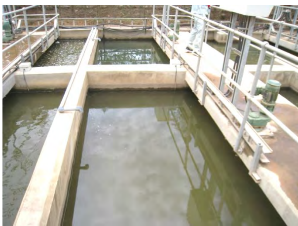
Figure 6-1 Result of Trial for Water Quality Improvement in Toker WTP (Flocculation Basin Left: before Trial, Right: after Trial)
