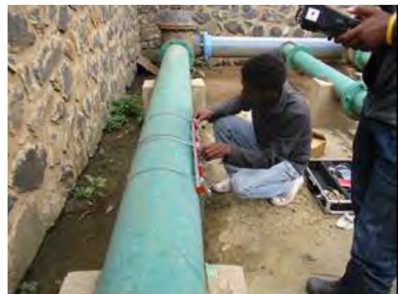
Figure 3-8 Training of Installation of Water Flowmeter
