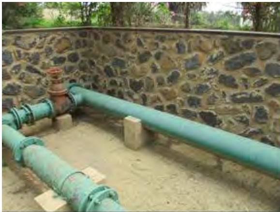
Figure 3-7 Example of Metering Point of Water Flow (Left: Inlet of S.V. WTP; Right: Outlet of New Sembel Pump Station)
