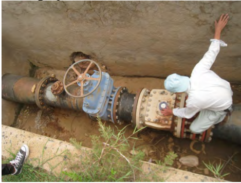
Initial Joint Investigation
