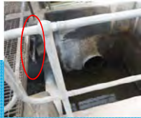
Inlet Channel from Tokor Dam
