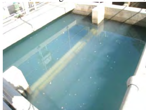
Trial of Water Quality Improvement in Toker WTP (Flocculation after Cleaning: The difference of water color is observed.)
