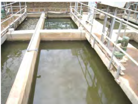
Trial of Water Quality Improvement in Toker WTP (Flocculation before Cleaning)
