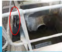
Inlet Channel from Tokor Dam
