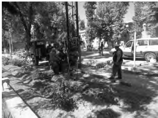
Shaft-sinking and tunneling works
