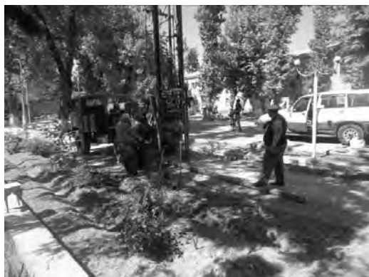
Shaft-sinking and tunneling works
