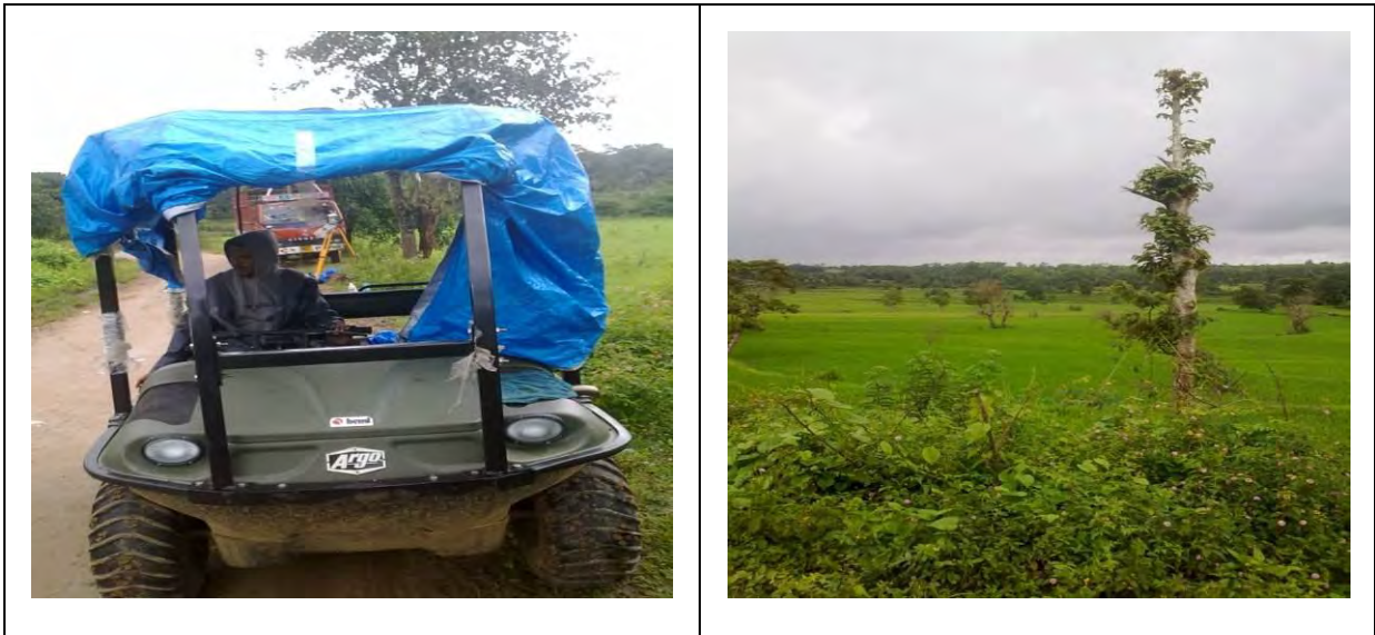
Images Showing Base station setup on the Control point GPS24 and Mobile lidar equipment Mounted on 6X6 Argo vehicle and initiation of survey, paddy fields near the alignment
