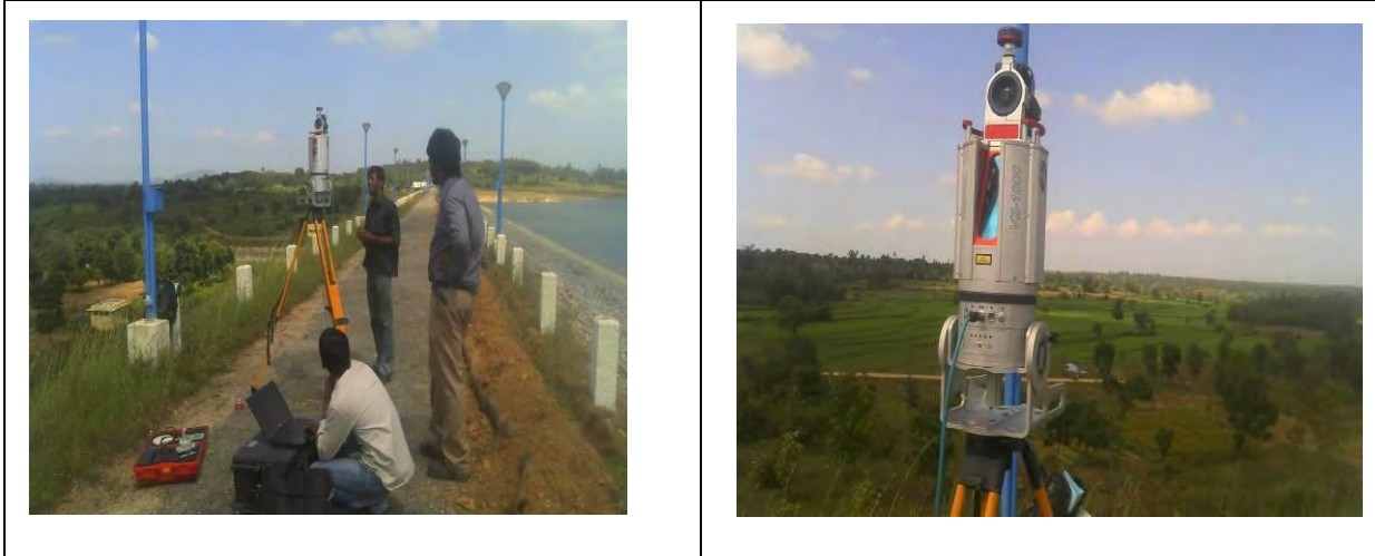
Images showing testing and survey using Terrestrial Scanner on top of Vate hole Dam
