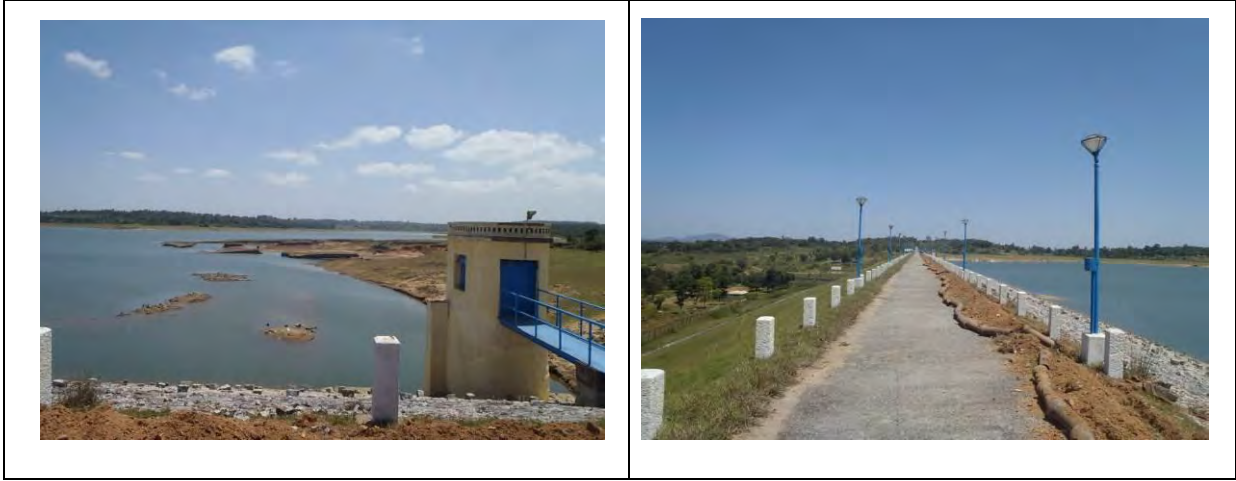
Images Showing the Vate Hole Dam and topography of the surrounding location
