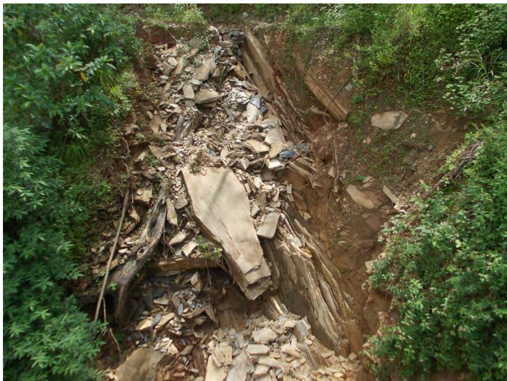
Figure 12 : Schist outcropping near km 12500
