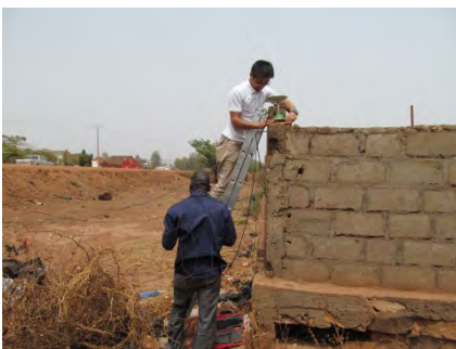
Training on GNSS Antenna Installation
