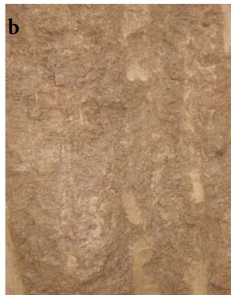
Figure 2. a) 15 test-pit 1 b) wall of test-pit 1
