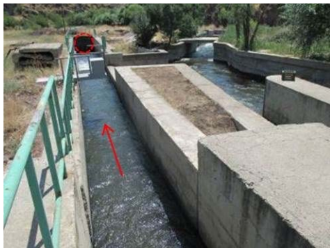
Figure A-25 Intake of Thakahan Canal (No.1)
