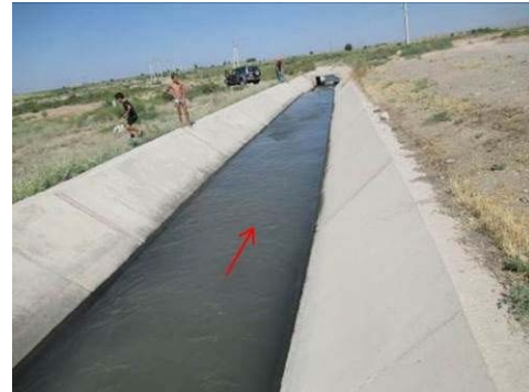
Figure A-93 Metsamor Canal (Main Canal) (No.2)
