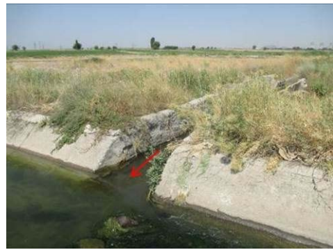
Figure A-87 Diversion from Lower Hrazdan Canal (No.8)
