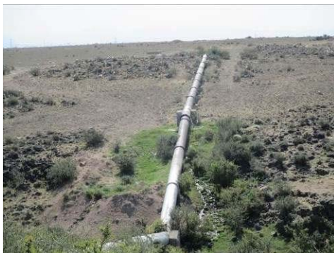
Figure A-29 Siphon (φ1200mm) (No.30)
