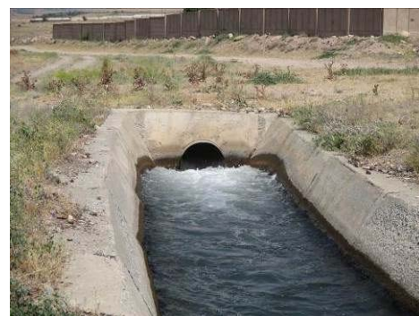
Figure A-6 Outlet of pipe from Arzni-Shamiram Canal to Arzni Branch Canal
