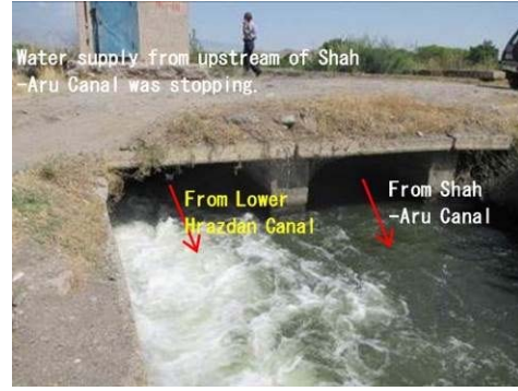
Figure A-49 Diversion from Lower Hrazdan Canal (No.4)
