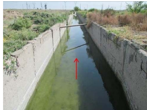
Figure A-76 Inner Aknalich Canal (No.2)
