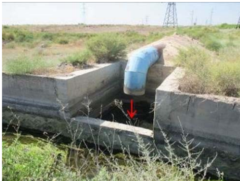
Figure A-70 Diversion from Lower Hrazdan Canal (No.6)
