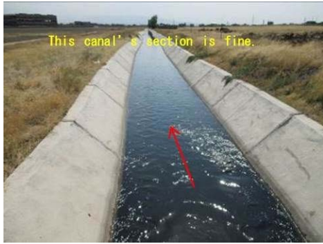
Figure A-13 Upstream of Canal under Control of Yeghvard WUA (No.4)
