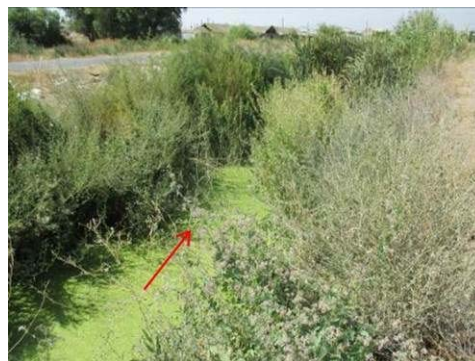
Figure A-85 No Used Canal (No.23 )
