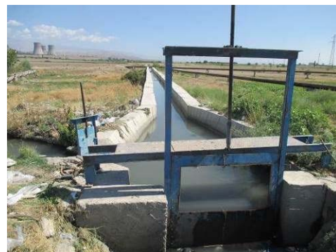
Figure A-102 Diversion from Lower Hrazdan Canal (No.6)
