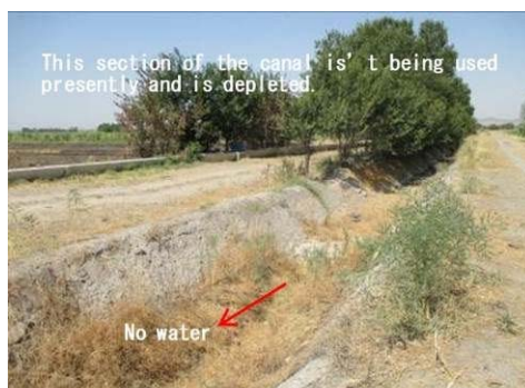
Figure A-58 No used Downstream Canal (No.34)
