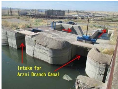
Figure A-1 Intake of Arzni-Branch Canal (No.1)
