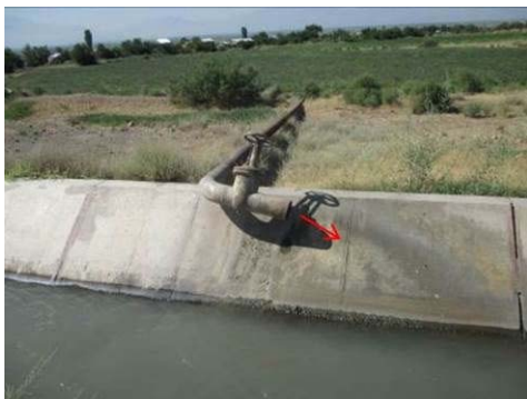
Figure A-101 Outlet of Pipe ( \phi 220mm) from Metsamor PS (No.2)
