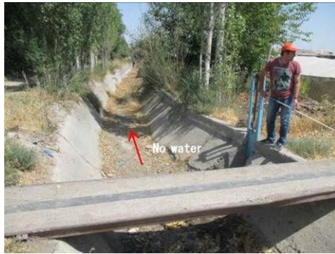
Figure A-79 No Used Canal (No.21)
