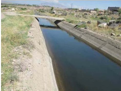
Figure A-31 Upstream of Canal (No.9)
