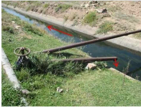
Figure A-36 Outlet of Pipe( \phi 200mm)
