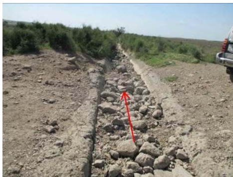
Figure A-8 Connection Canal to Thakahan Canal (No.42 )
