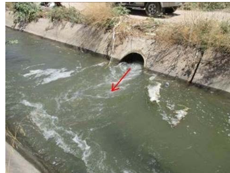
Figure A-71 Diversion from Lower Hrazdan Canal (No.25)
