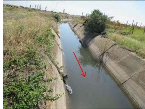
Figure A-29 Upstream of Canal (No.19)
