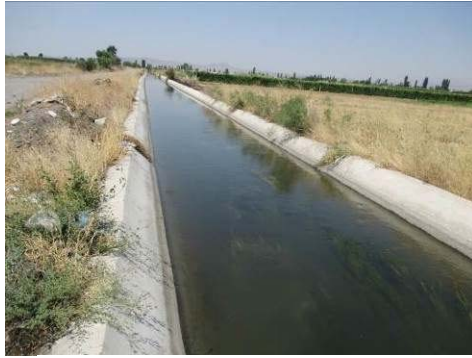
Figure A-40 Shah-Aru Canal (No.13)
