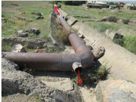
Figure A-24 Outlet of Pipe ( \phi 500\text{mm} ) (No.40)
