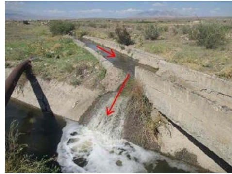
Figure A-37 Diversion from Arzni- Branch Canal (No.22)
