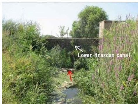
Figure A-41 Under pass to Cross Lower Hrazdan Canal (No.4)
