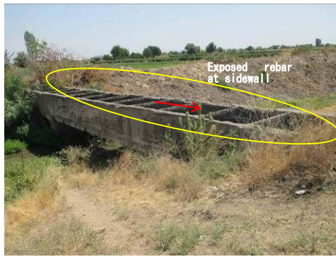
Figure A-54 Aqueduct Bridge (No.23)
