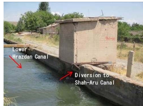
Figure A-42 Diversion from Lower Hrazdan Canal (No.4)
