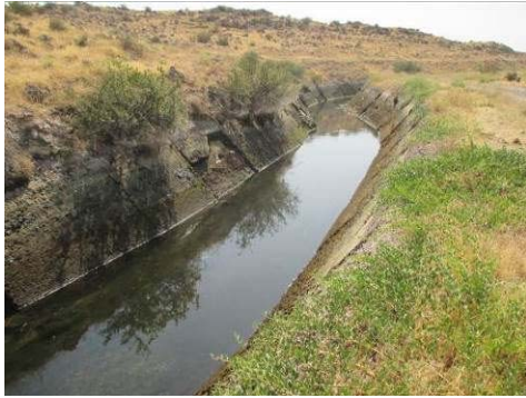
Figure A-115 Crack of Side Wall (No.27) Figure A-116 Shortage of freeboard of Side Wall (No.23)
