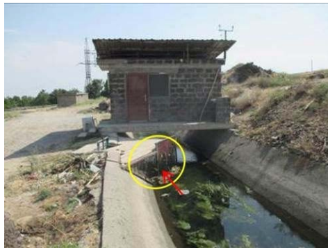
Figure A-114 Diversion to Upper Aknalich Canal (No.64 )
