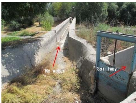
Figure A-77 Aqueduct Bridge (No.20)
