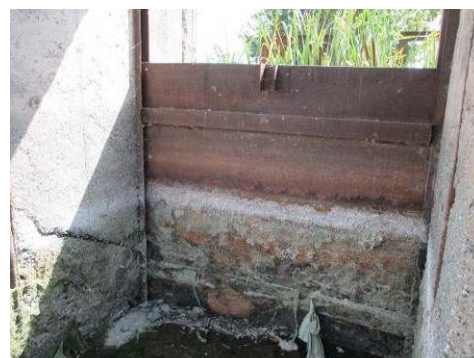
Figure A-63 Inlet of Pipe to Inner Aknalich Canal (No.2)
