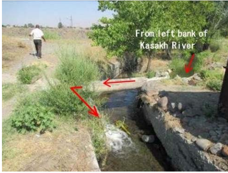
Figure A-48 Diversion of Water of Kasakh River that Detour to Left Bank (No.2)
