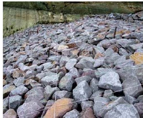
Figure 6-5-6.4 Example of Rock Rip Rap
