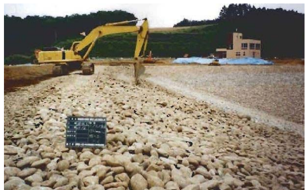
Figure 6-5-6.7 Example of Cobble-Gravel Rip Rap
