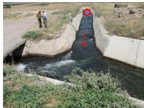
Figure 4-4-4.4 Outlet of Pipe from Arzni-Shamiram Canal (ø800mm) (Arzni-Branch Canal at No.25)
