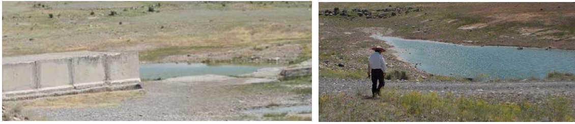
Figure 4-3-6.5 Ponds on the Reservoir Bottom at the Upstream of Dam-No.1
