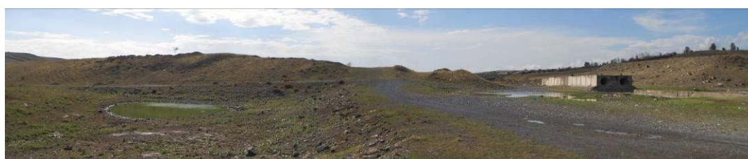
Figure 4-3-7.1 Existing Dam Body (Dam No.1)
