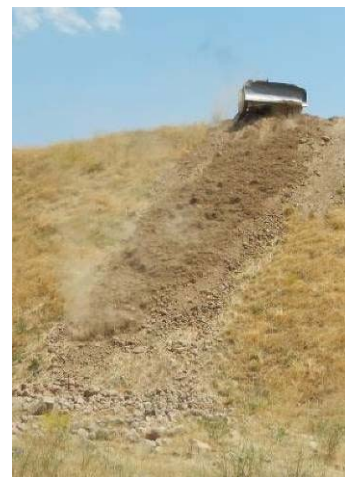
Figure 4-3-4.7 Segregation through Falling
