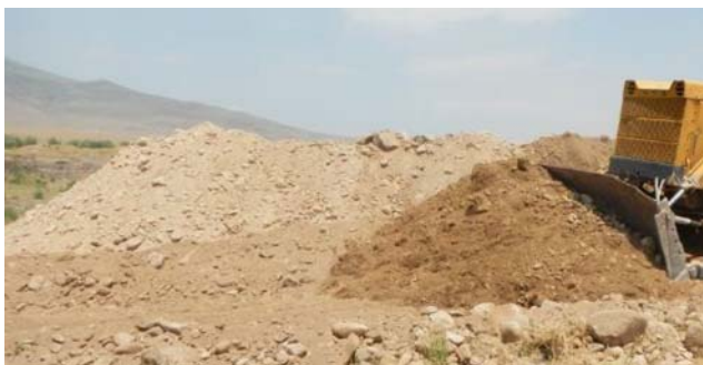
Figure 4-3-4.6 Mounded Sand-and-Gravels after Excavation
