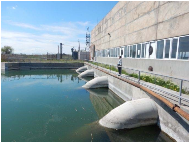
[Photo-9] Ranchapar Pump Station
