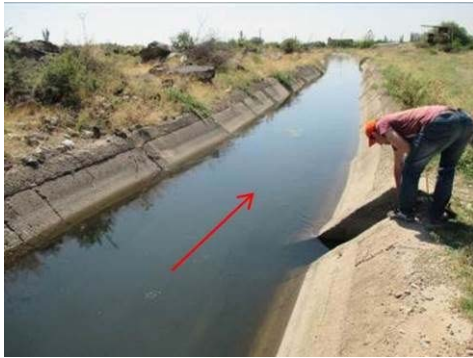
Figure A-27 Thakahan Canal (No.6)
