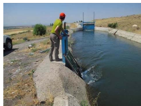
Figure A-4 Intake of pipe from Arzni-Shamiram Canal to Arzni Branch Canal
