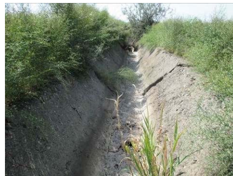
Figure A-9 Connection Canal to Thakahan Canal (No.42 )
