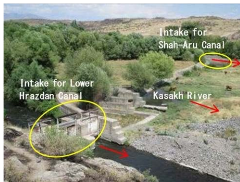
Figure A-38 Kasakh Weir (No.1)
