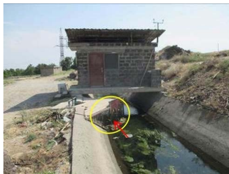
Figure A-114 Diversion to Upper Aknalich Canal (No.64)
