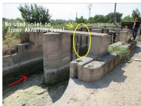
Figure A-62 Inlet of Pipe to Inner Aknalich Canal (No.2)
