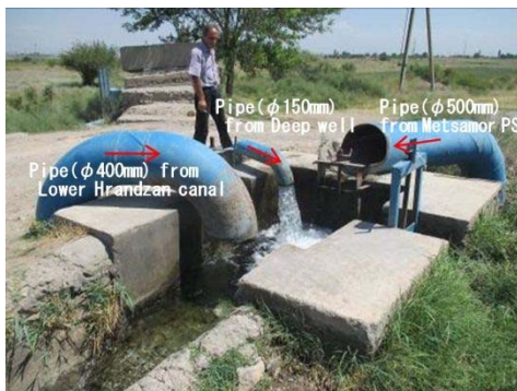
Figure A-94 Outlet of Pipe ( \phi 500\text{mm} ) from Metsamor PS (No.25)
