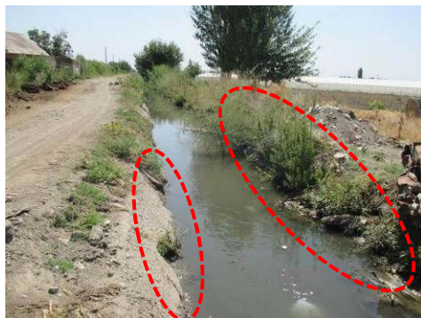
Figure A-66 Depleted Sidewall (No.29)
