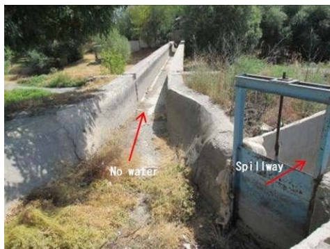
Figure A-77 Aqueduct Bridge (No.20)
