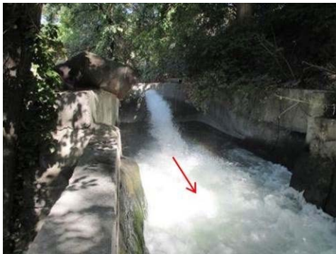
Figure A-75 Outlet of Pipe ( \phi 1,000\text{mm} ) from Aknalich PS (No.1)
