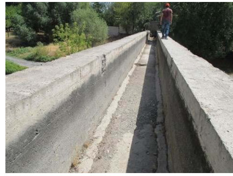
Figure A-80 No Used Aqueduct Bridge (No.20)
