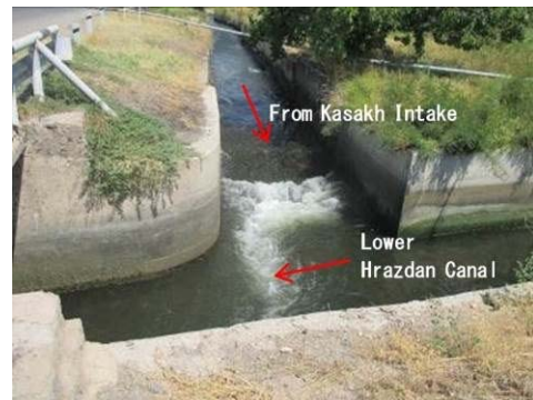
Figure A-118 Diversion from Kasakh Intake
