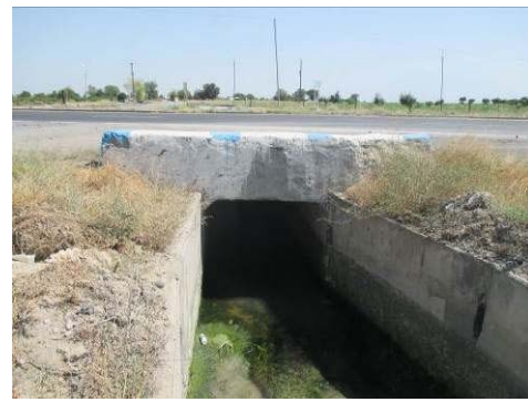
Figure A-55 Crossing Point of Road (No.13)
