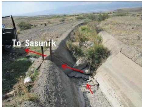
Figure A-7 End of using canal (No.33 )
