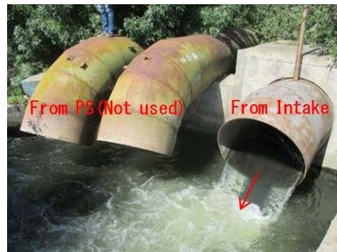
Figure A-26 Outlet of Pipe ( \phi 1500\text{m} ) from the Intake (No.3)
