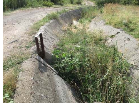
Figure A-19 Disused Canal not Used (No.35)
