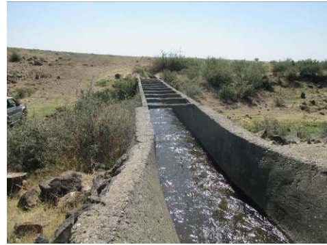
Figure A-28 Aqueduct Bridge (No.38)
