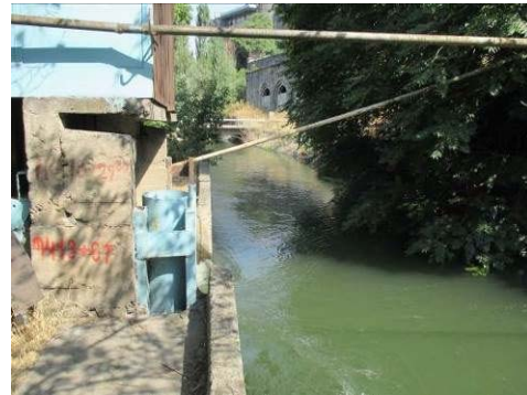
Figure A-106 Intake for Lower Hrandzan Canal (No.2)
