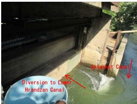
Figure A-107 Intake for Lower Hrandzan Canal (No.2)
