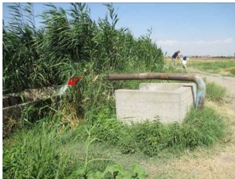
Figure A-50 Outlet of Pipe from Deep (No.27)
