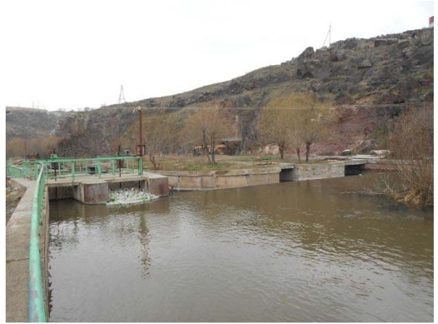
[Photo-8] Takahan Intake
