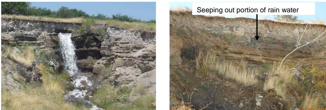
Figure 4-3-6.6 Conditions Observed on the Cliff Slope of Sand-and-Gravels
