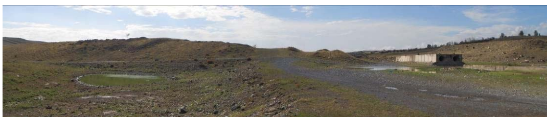
Figure 4-3-7.1 Existing Dam Body (Dam No.1)
