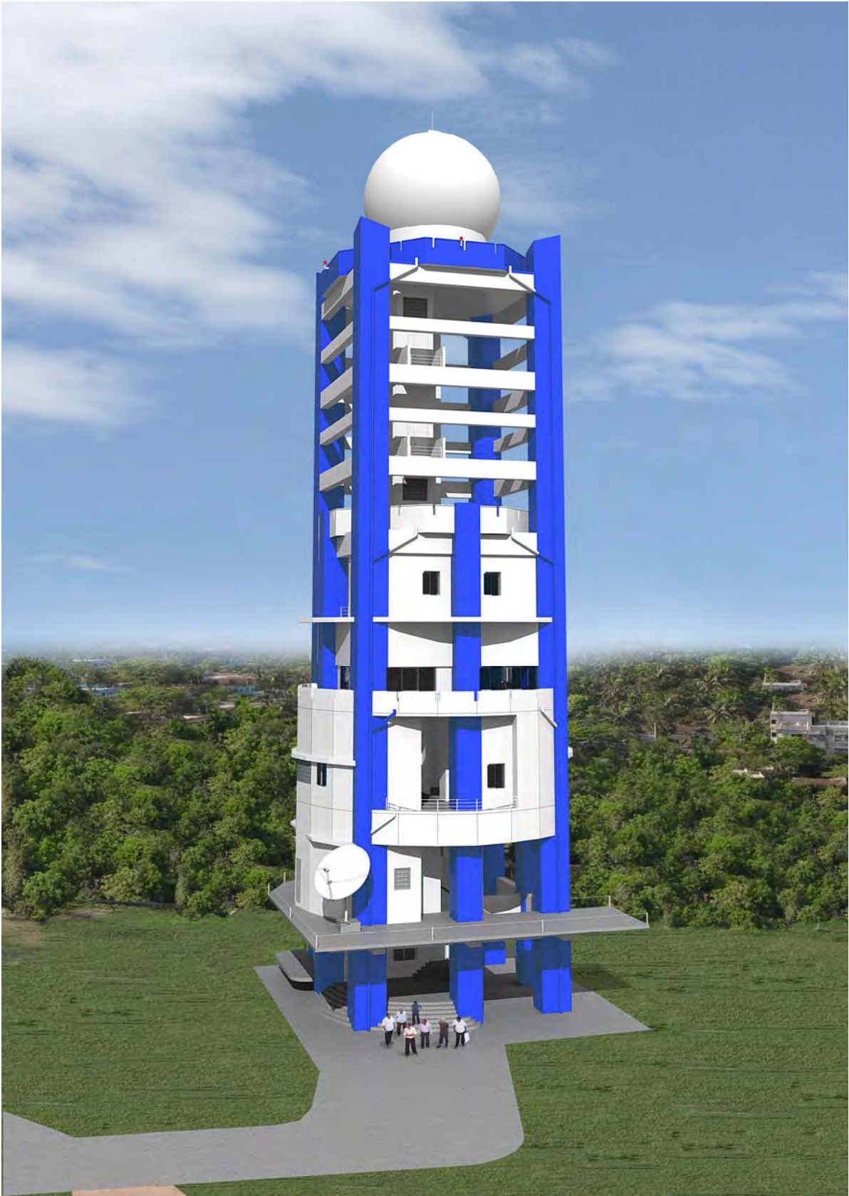
Puttalam Meteorological Radar Tower Building
