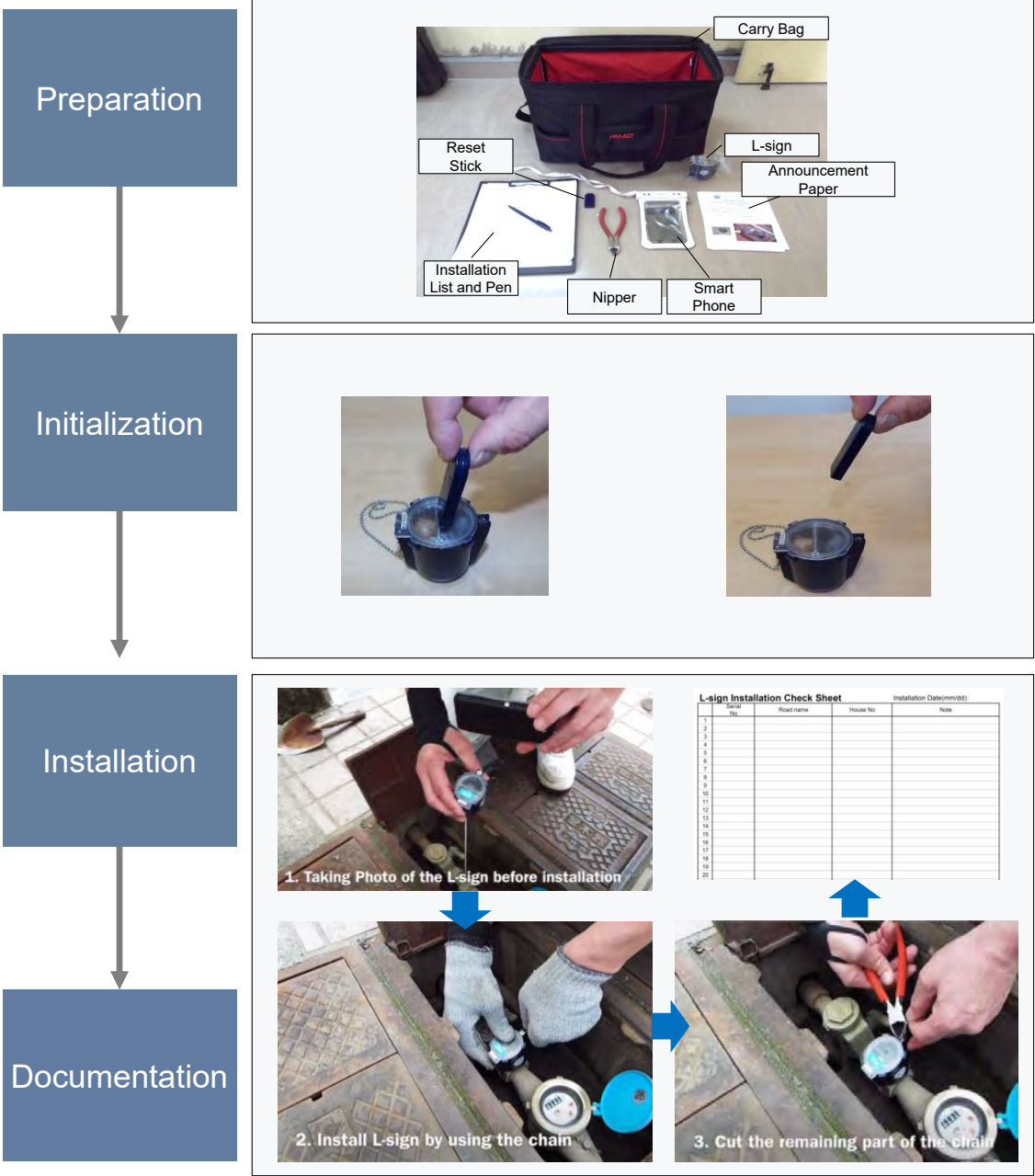
Figure 3-11 L-sign for supply pipe installation flow
