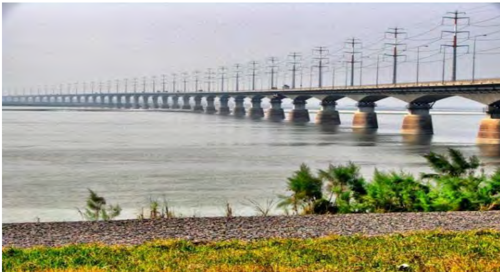
Figure 8.1 Bangabandhu Multipurpose Bridge
