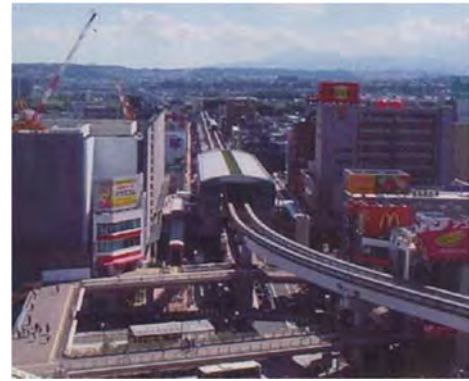
Sub-center development at a railway station in Tokyo.
