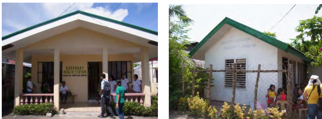
Figure 5- 5 Barangay Health Station in Camarines Sur
