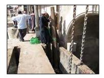
Picture: A situation of the closing gate (hit on the gate with wood)
