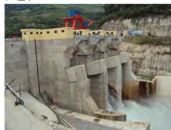
NamKhan Dam3 HPP
