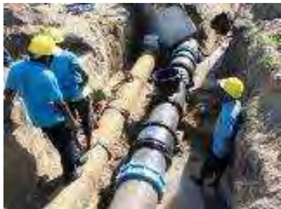
Output-4 (Leakage Management): the 3rd Year Fieldwork of pilot project came to the most important portions such as branch connection of primary pipelines. During this inserting work period of 5 hours, water supply from Saateni Elevated tank is suspended.
