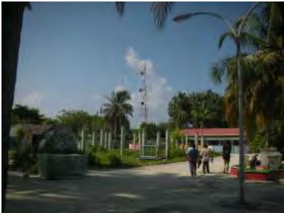
Outer circumference of the site where antenna tower to be built in Guraidhoo
