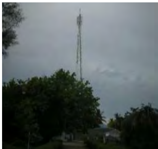
Outer circumference of the site where antenna tower to be built in Hithadhoo
