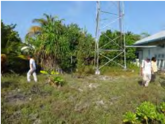
Existing station building and antenna tower at the site in Kulhudhuffushi
