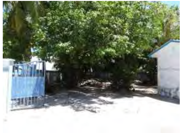
The site where antenna tower to be built in Ungoofaaru
