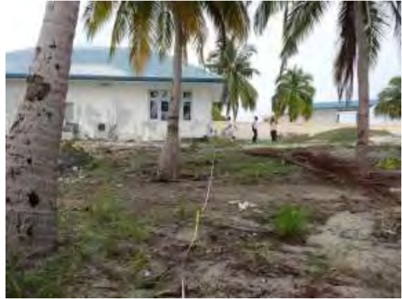
The site where antenna tower to be built in Dhidhdhoo
