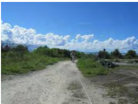
The site where antenna tower to be built in Thinadhoo
