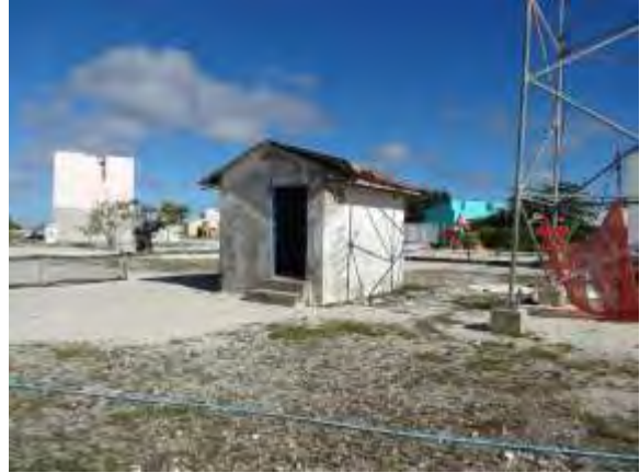
Existing station building at the site in Naifaru
