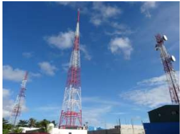
Antenna tower of telecom carriers at the site in Malé (Villingili)
