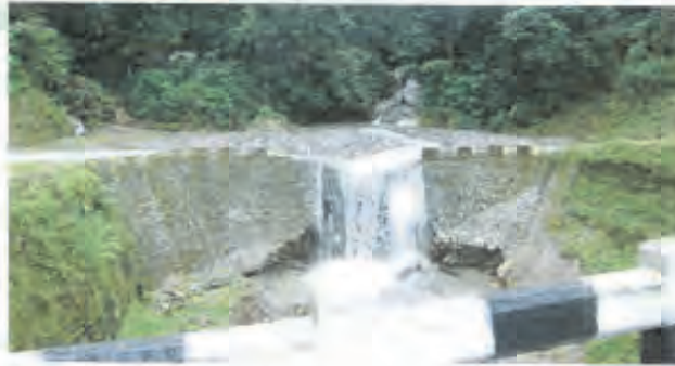
Figure-5 Temporary detour at upstream of Beteni Bridge (during monsoon)
