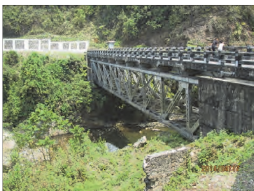
Samkhara Bridge : Steel Truss Bridge Length 61m, Width 4.3m Construction: Year 2001
