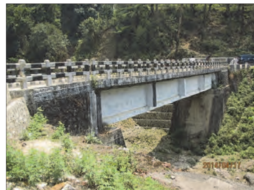
Beteni Bridge : RC-T Girder Bridge Length 25m, Width 4.2m Construction: Year 1987
