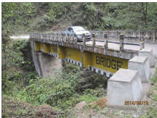
Telegangchu Bridge : RC-T Girder Bridge Length 25m, Width 4.5m Construction: Year 1981
