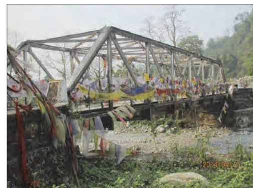
Passang Bridge : Steel Truss Bridge Length 40m, Width 7.5m Construction: Year 1970
