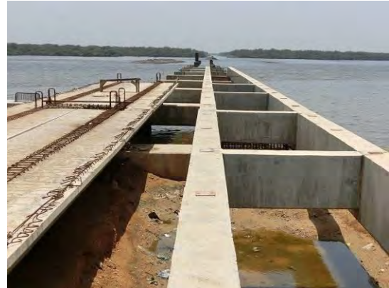
Photo 5.3-8: 2.5 km Trestle under Construction
