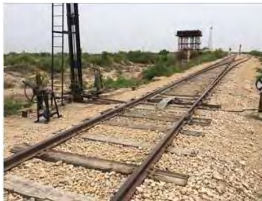
Figure 2-27 Mechanical Point at Budapur Station
