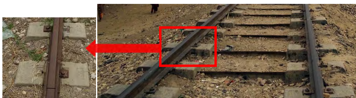
Figure 2-11 Typical RC Twin Block Sleeper
