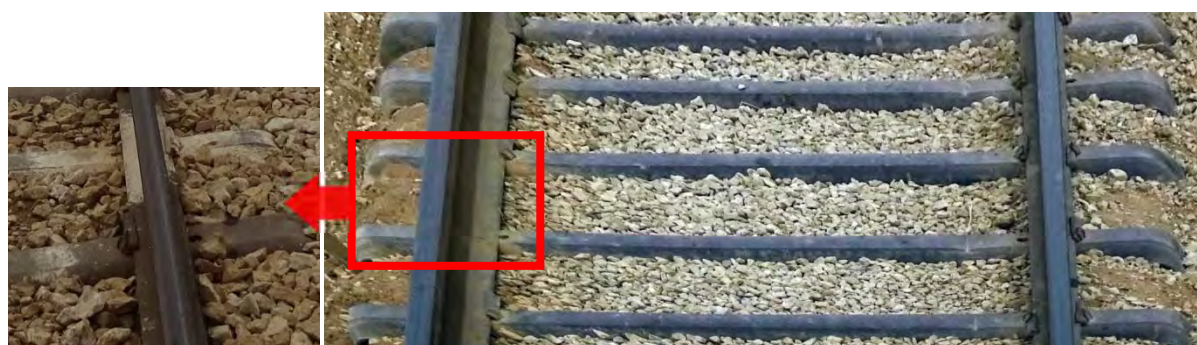
Figure 2-10 Typical Steel Sleeper
