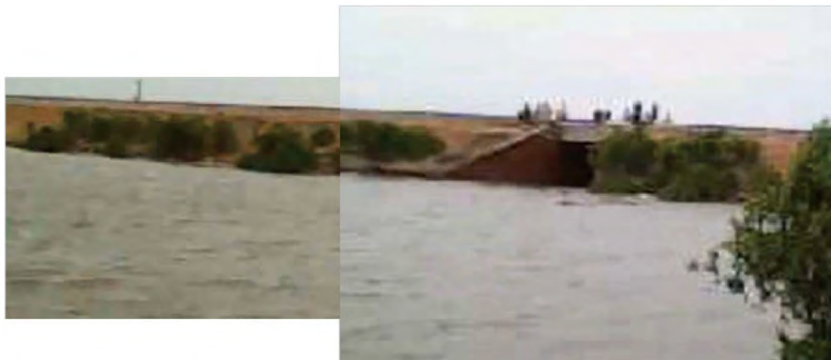
Figure 11-20 Erosion of Railway Embankment near Cadet College Petaro Station
