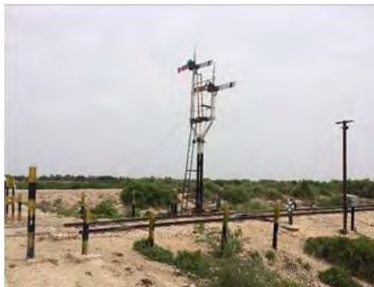
Figure 2-26 Mechanical Home Signal at Budapur Station
