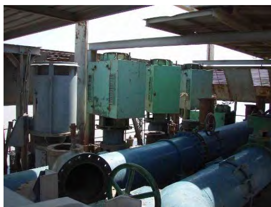
Photo 3.3-23 Pumps in Intake Tower-1
