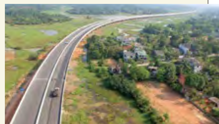
The outer circular highway just before opening in September 2015.
