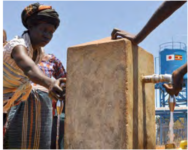
People in northern Uganda use the water supply equipment completed with Japanese Grants.
