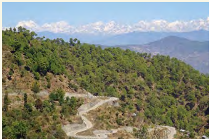
The Sindhuli Road meanders through the Mahabharat Range, with the Himalayas in the background. (Photo: Nippon Koei Co., Ltd.)
