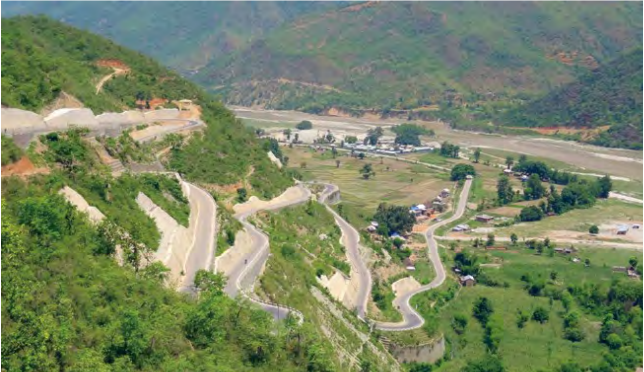
Sindhuli Road in Nepal. Construction progressed under Grants from 1995 and was completed after approximately 20 years. The road was functional even after the Nepal Earthquake in 2015, and became a vital transportation route for relief supplies.
