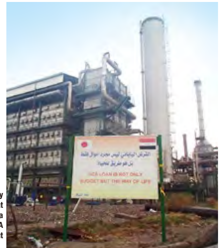
Iraq: A signboard placed by the maintenance agency at the rehabilitation site of a fertilizer plant says "JICA Loan Is Not Only Budget But Way of Life."
