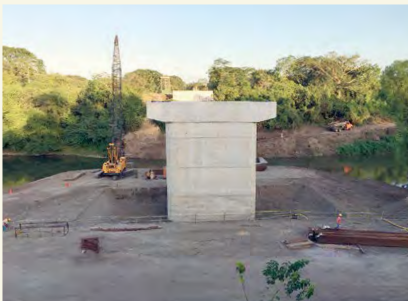
Paso Real, the 25th bridge being built under cooperation from Japan
