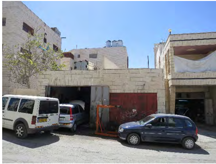
Sample Photo-3 ( right ) Industrial Building (Automobile mechanical garage)
