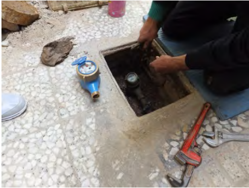
Replacing a Malfunctioning Meter
