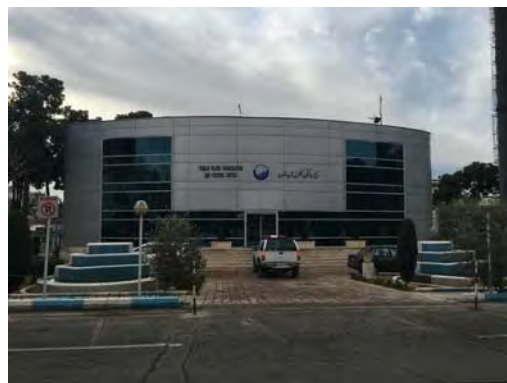
TPWWC Control Center
