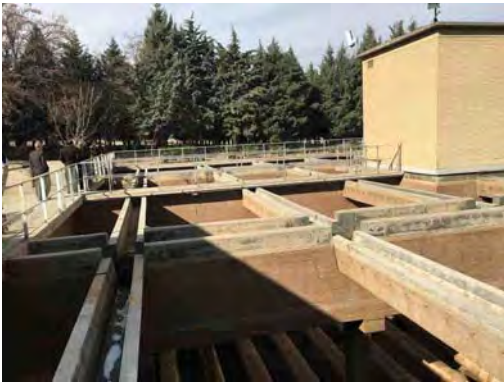
Water Treatment Plant No. 1
