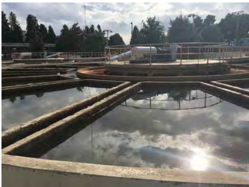
Jalailah Water Treatment Plant
