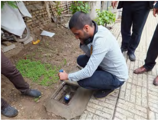
Water Leak Detection at House Connection
