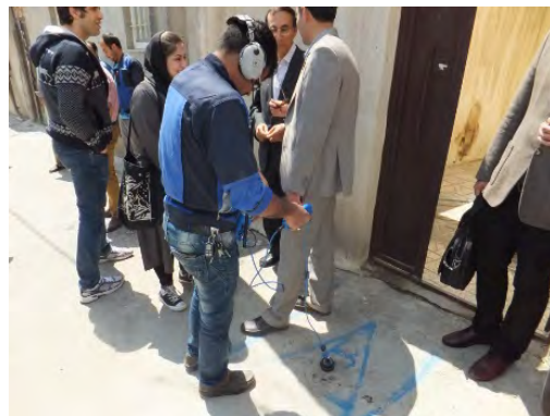
Detecting the Leaking Point
