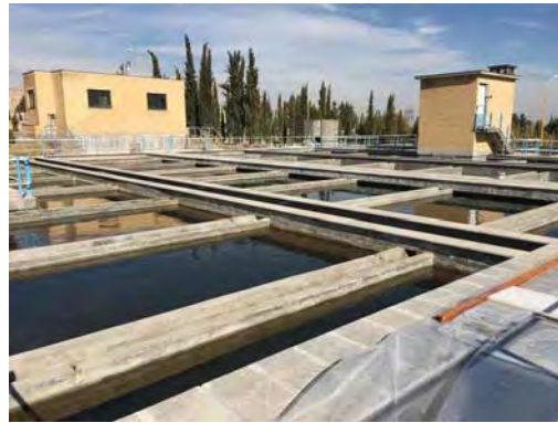
Water Treatment Plant No. 2
