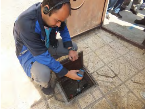
Water Leak Detection at a House Connection
